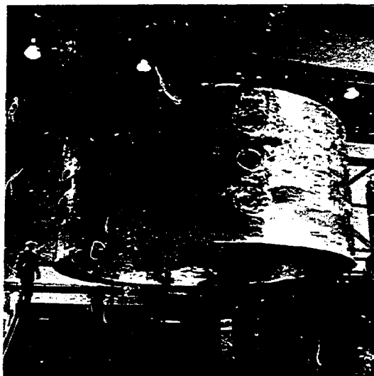
The world's largest superconducting magnet being installed in a new 148-inch bubble chamber at Argonne National Laboratory in Illinois.
